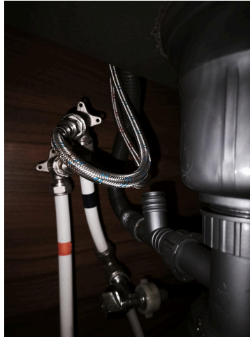
Kitchen tap connection
